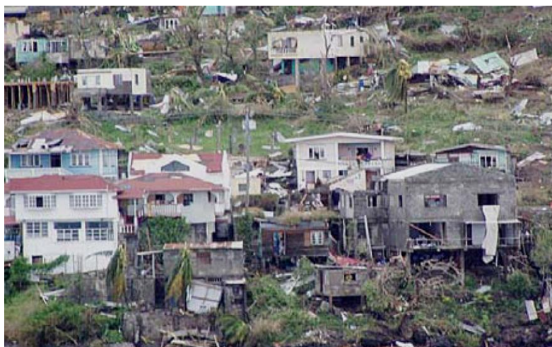
Figure 8: Housing damage from Hurricane Ivan, 2004 xiii
