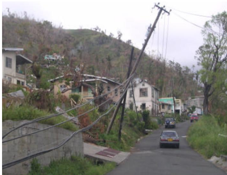
Figure 4.7.2: Public utility impacts resulting from Hurricane Ivan
