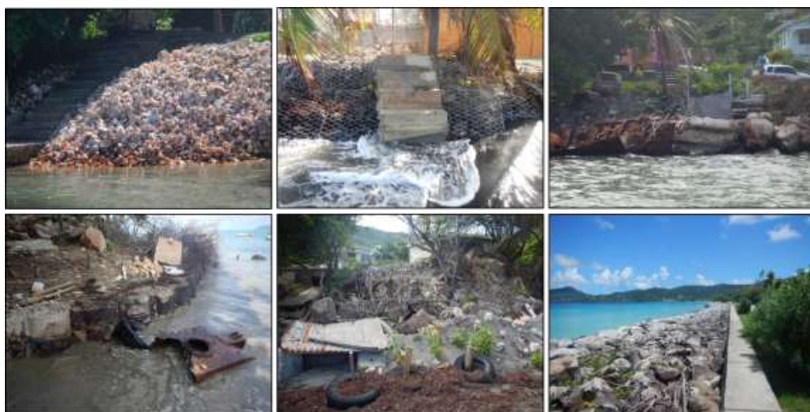
Figure 75-Coastal erosion at Windward in Carriacou and examples of shoreline protection structures used on the island of Carriacou ranging from conch shells to engineered armoured structures: Source (Day, Van Proosdij, Campbell, Lee, Baker, & Thomas, 2015)
