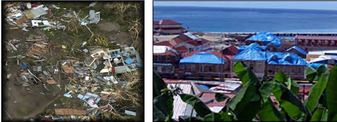
Figure 5.2: Showing tarpaulin roof on buildings after hurricane Ivan (Grenada)
