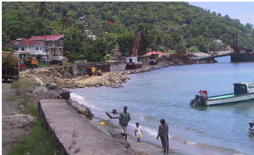
Figure 4.8: Coastal construction post hurricane Lenny, South-west coast Grenada
