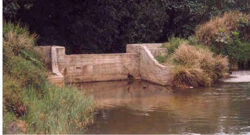
Figure 3.12a: A typical weir that can be used to increase on-river storage in Northern Grenada
