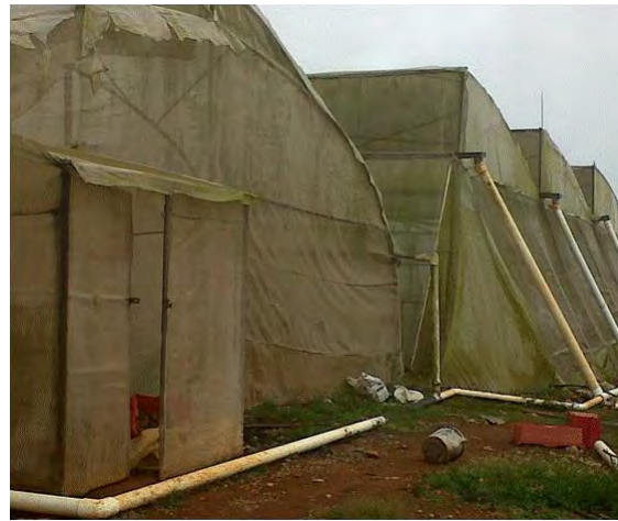
Tarpaulin RWH from greenhouse (Jamaica)
