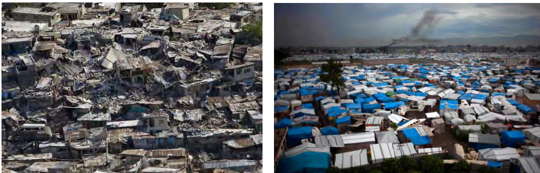
Figure 5.3: Haiti 2010 earthquake aftermath
