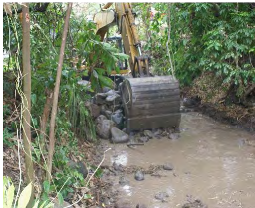
Figure 3.12b: River clearing to increase on-river storage in Northern Grenada
