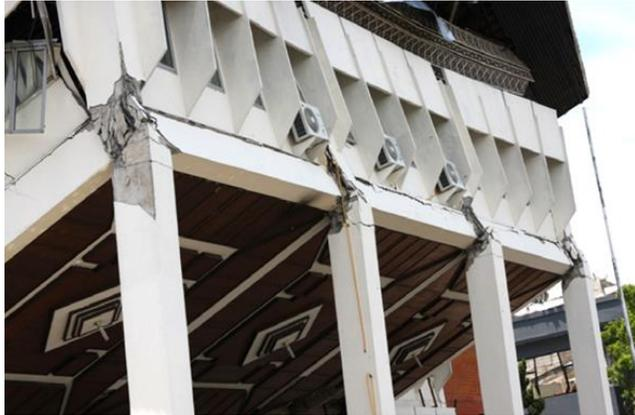
Fig 2 – Load path failure
