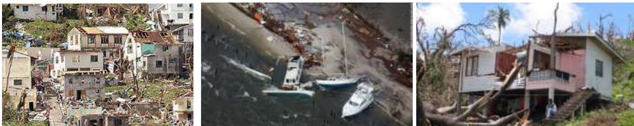
Damage from Hurricane Ivan
