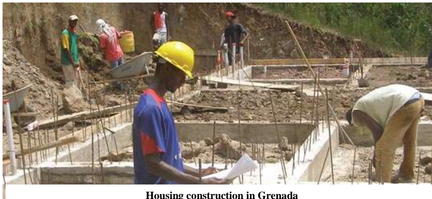
Housing construction in Grenada
