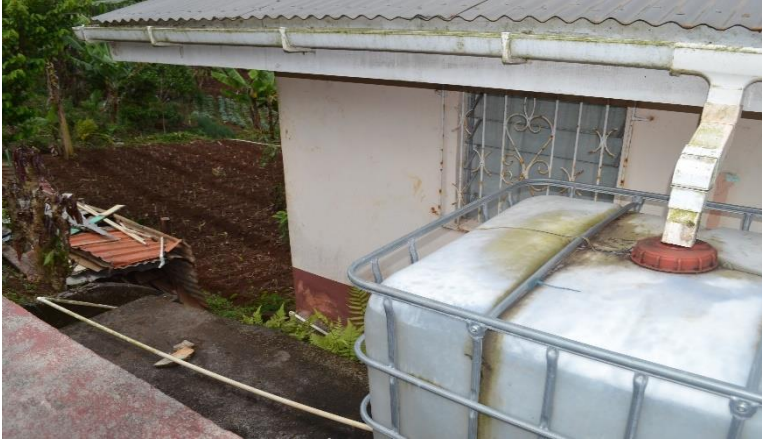
Rain Water Harvesting for irrigating a farm in Mardi Gras, St George
