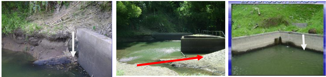
Figure 3-47: Drought of 2013 and reduced water level and siltation for Annandale (shown by arrow)
