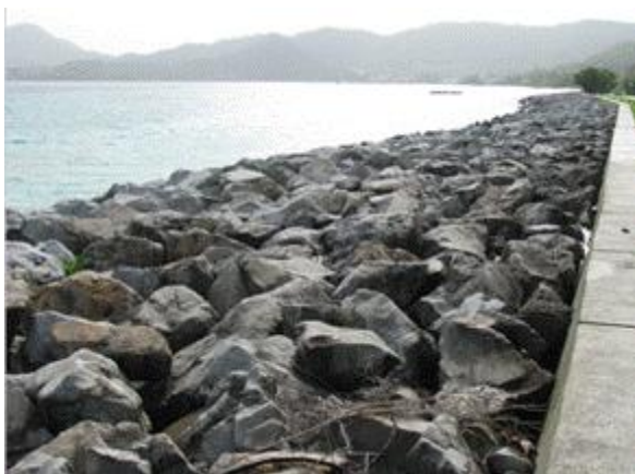
Figure 9.8: Protective sea wall and stone works mitigate the impact of erosion at Lauriston, Carriacou
