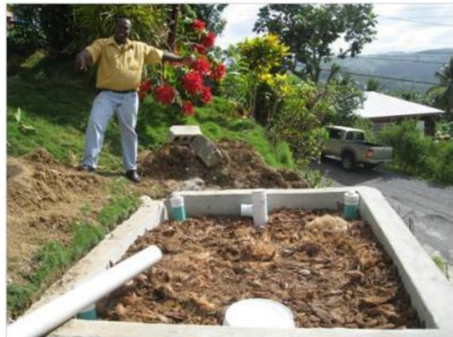
Figure 4.18: A small scale wetland infiltration system under construction
