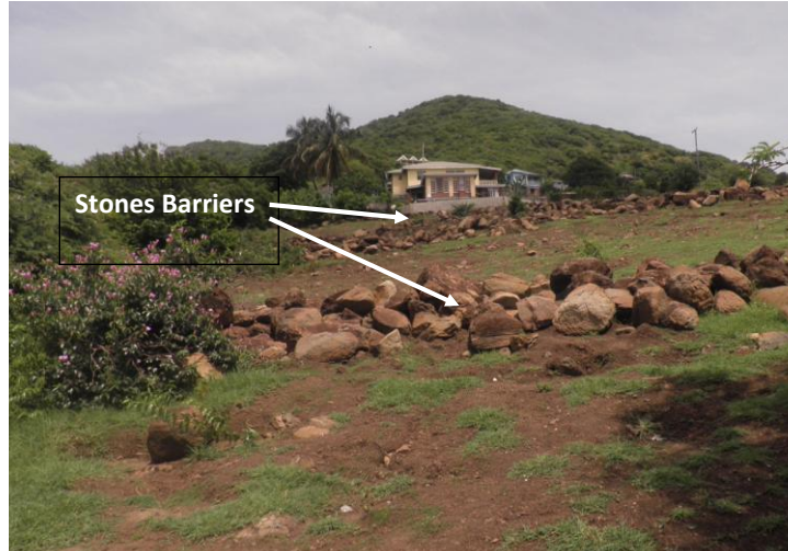
Figure 9.16: Stone barriers successfully established to reverse hillside erosion in Carriacou
