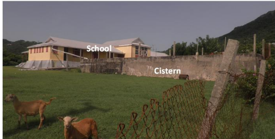
Figure 4.10: Communal cistern (roof catchment) at the Dover Government School, Carriacou.
