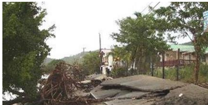
Figure 9.4: Beach erosion at Harvey Vale due to storm surges generated by Hurricane Lenny in 1999 leading to the collapse of a main roadway
